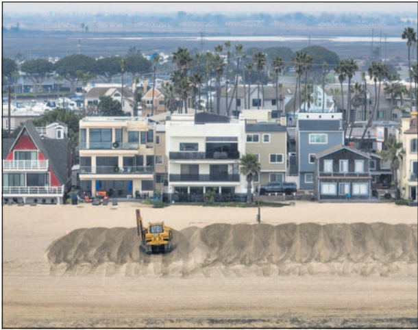
A heavy equipment operator builds a sand berm at Surfside in Seal Beach on Monday ahead of a strong storm forecast to arrive by the late evening.
